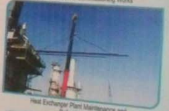
Heat Exchanger Plant Maintenance and Refurbishment
