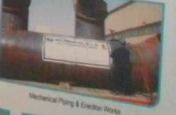
Mechanical Piping & Erection Works
